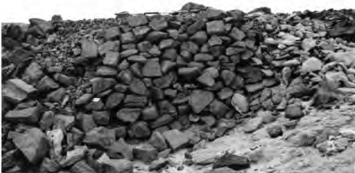
Figure 13.3: Detail of the main quarry road: two views of the embankment near quarry P.
